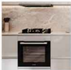
Stove, Exhaust Hood - Connected with main building extract/exhaust system. Built in Oven.
